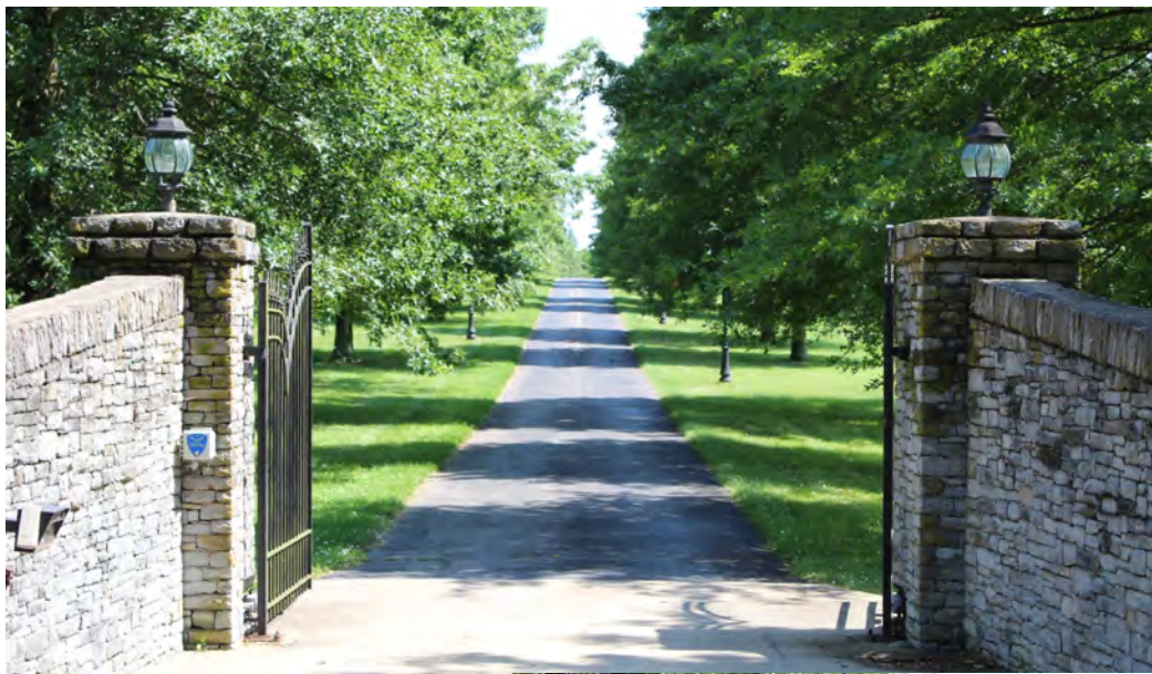
Stone entry with electronic security gate
