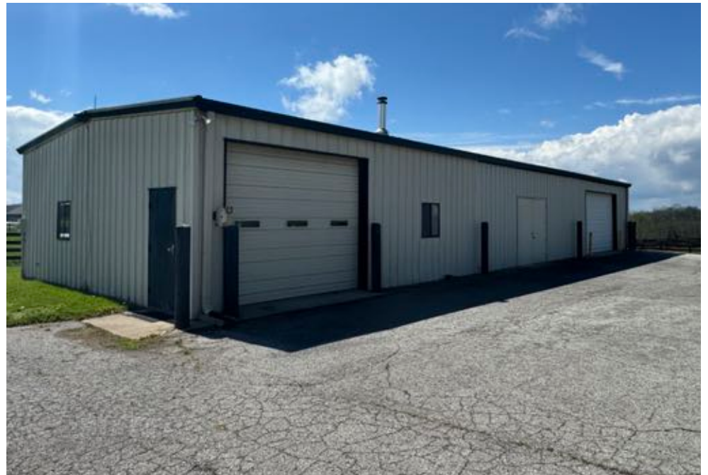
Aquatred and cold water spa dedicated building
