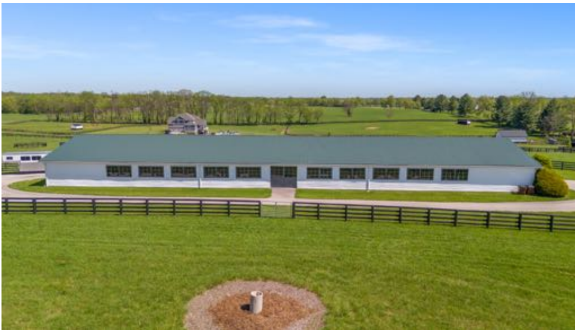
View of Barn 2 with new roof and new windows
