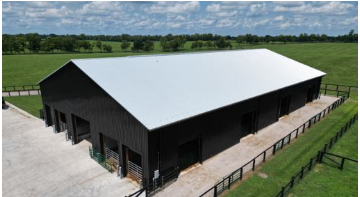
84x145 cattle penned feed barn with 18' aisle, 16' roll up door and 14' roll up doors around the exterior
