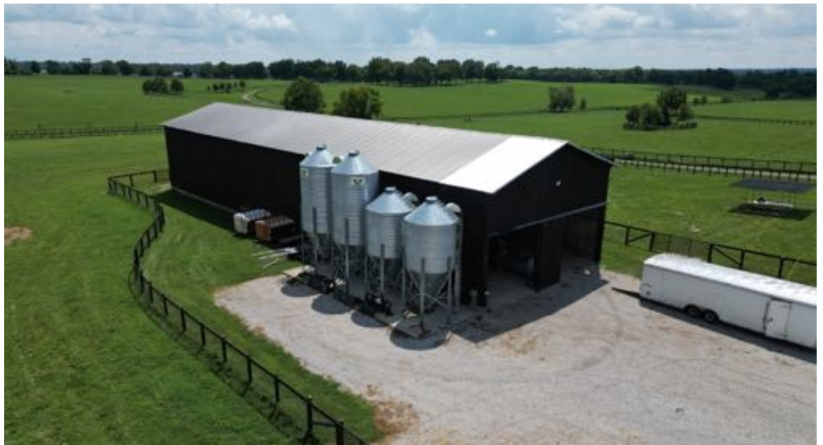
142x38 equipment and hay storage barn with 4 stainless steel grain bins and unloader
