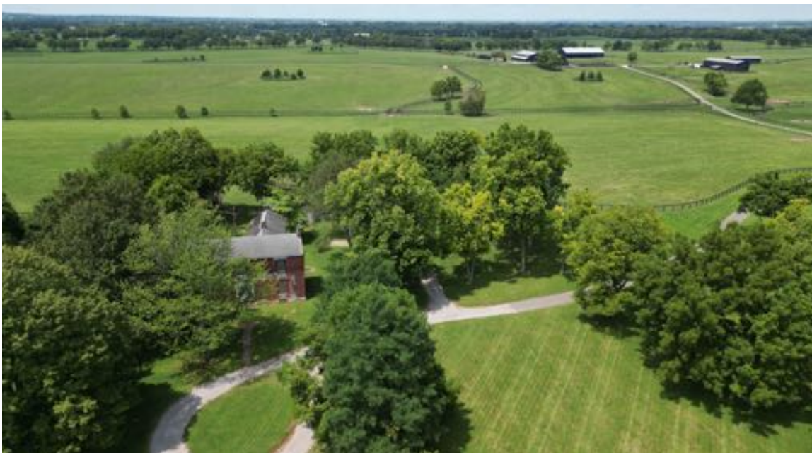
Historic residence in need of renovation
