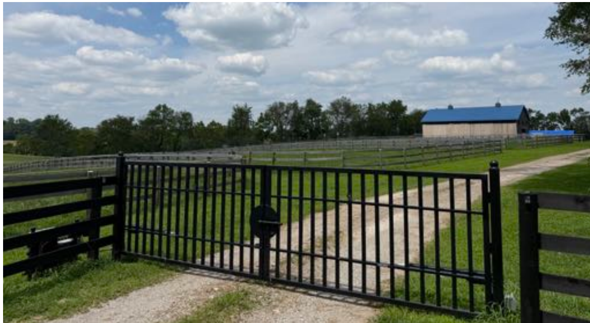
Automatic gated entry to barn
