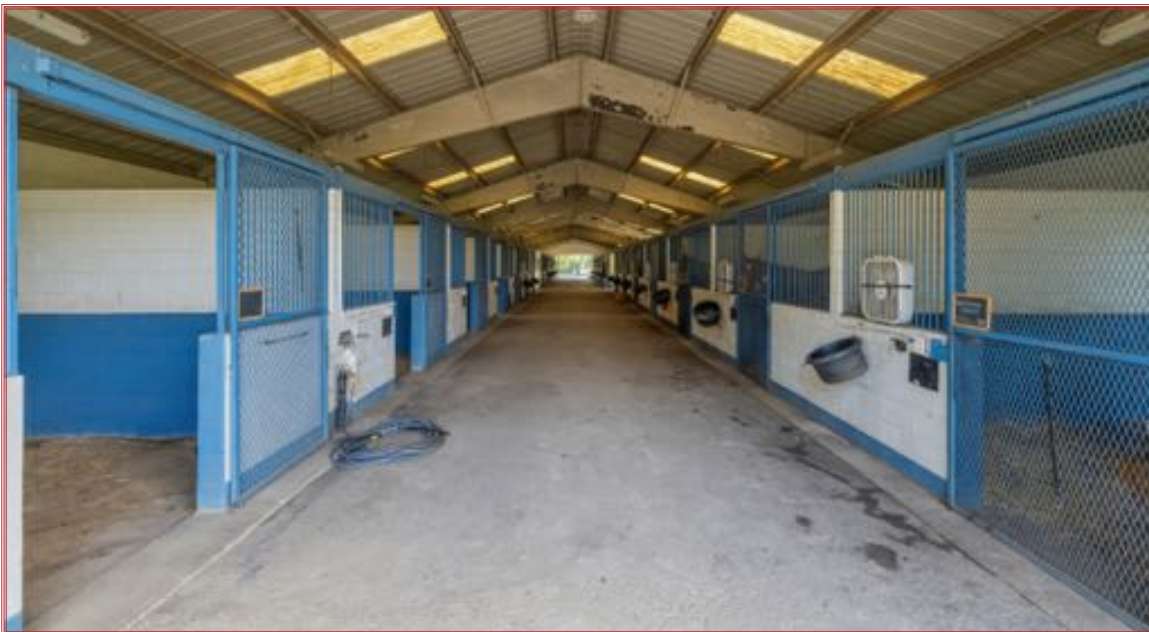
Barn C 27 stall concrete barn with 14' x 14' stalls, tack room, lab and wash area
